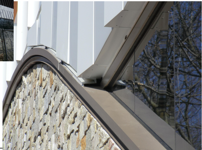
Curved stone with curved CMU back-up
