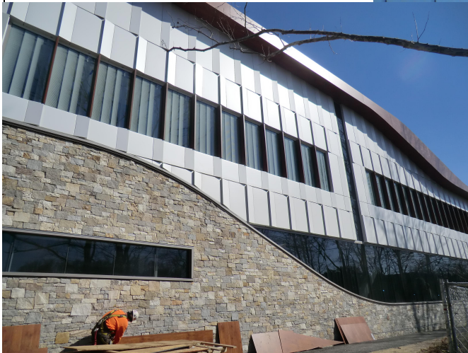
Curved stone with curved CMU back-up
