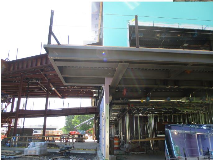
Patio Canopy Cantilevered steel
